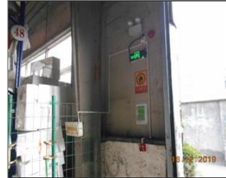
Photo of fire safety equipment Fire alarm Emergency lamp and Exit sign.JPG
