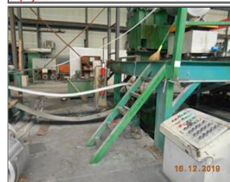
Photo of non-conformity NC7.17 No handrail was installed for the ladder.JPG
