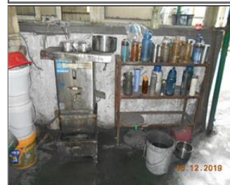
Photo of the sanitary facilities Drinking water.JPG
