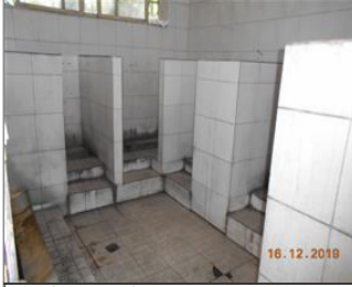
Photo of the sanitary facilities Toilet.JPG
