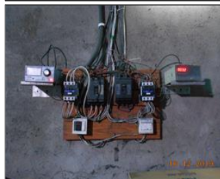
Photo of non-conformity NC7.13 The power switch was exposed and installed on the wooden board.JPG
