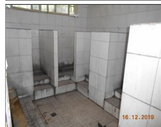
Photo of non-conformity NC7.22 No private door was installed for the toilet.JPG
