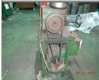
Photo of non-conformity NC7.17 No safe guard was installed for the belt of the machine.JPG
