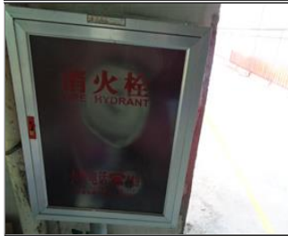
Photo of fire safety equipment Fire hydrant.JPG
