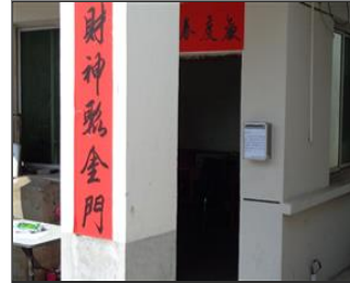
Photo of non-conformity NC-Suggestion box was installed at security guard room could not protect privacy.JPG
