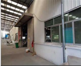
Photo of the inside of the main production hall Building rented to a vacuum cup factory.JPG
