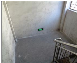
Photo of fire safety equipment Staircase with evacuation indication sign.JPG
