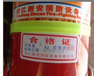
Photo of fire safety equipment Certificate of approval for fire extinguisher.JPG
