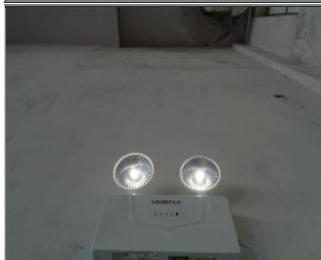
Photo of fire safety equipment Emergency light worked normally.JPG
