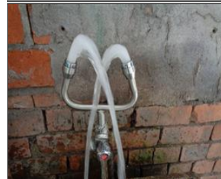
Photo first aid facilities Eye washing station.JPG
