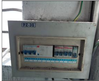
Photo of non-conformity NC-No outer cover for electrical switch box.JPG
