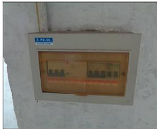
Photo of non-conformity NC-No electric shock warning sign on electrical switch box.JPG
