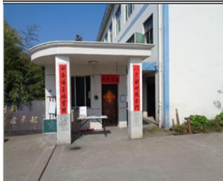
External photo(s) of the production unit(s) Security guard room.JPG
