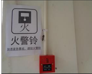
Photo of fire safety equipment Fire alarm trigger.JPG
