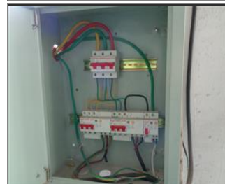
Photo of non-conformity NC-No inner cover for electricity distribution box.JPG
