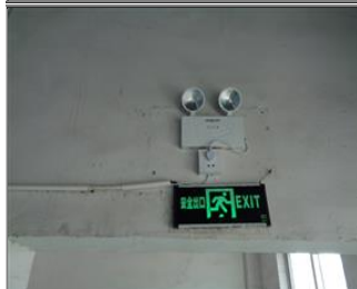
Photo of fire safety equipment Exit with emergency light and exit sign.JPG
