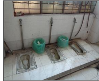
Photo of non-conformity NC-No private door or shield for toilet.JPG
