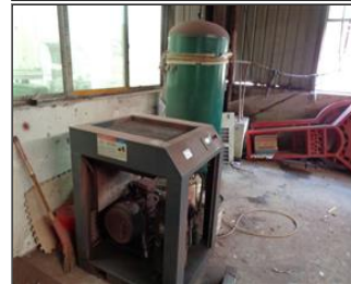
Photo of the inside of the main production hall Air compressor and simple pressure vessel.JPG
