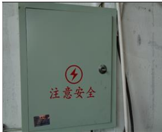
Photo of fire safety equipment Outside view for electricity distribution box.JPG
