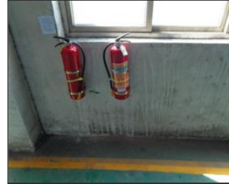
Photo of fire safety equipment Fire extinguisher.JPG
