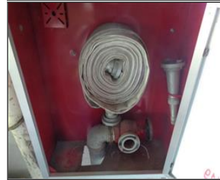
Photo of fire safety equipment Inside view of fire hydrant.JPG
