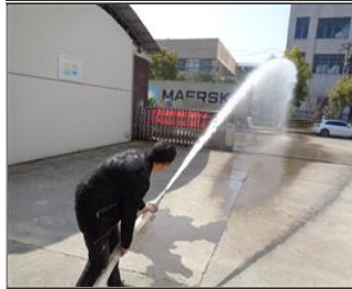
Photo of fire safety equipment Fire water with adequate pressure.JPG
